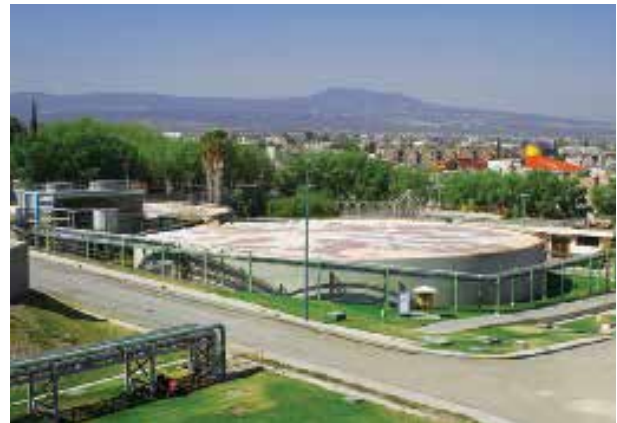
Wastewater treatment facilities at the Bajío plant
